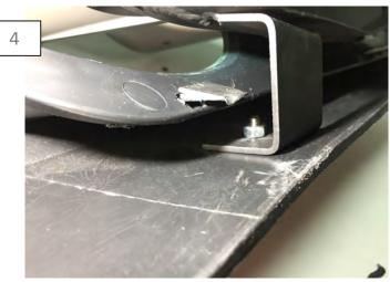
Install the Quad Tips using the supplied hardware. Place the screw through the diffuser so that the nut is on the hidden side of the diffuser. \*\*Note: Do not over tighten the screws. Doing so can pull the threads out of the bosses.
