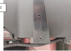
Using a drill and a 1/4" drill bit, drill (2) holes on each diffuser fin. \*\*Note: Be careful not to apply alot of pressure drilling upward.
