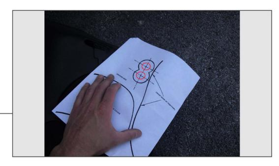
Using the provided template shown below, drill 1/8" pilot holes through each of the cross sections. Once the pilot holes are drilled through the panel, follow with a  $1\,3$ 4" hole saw through the outside of the panel. These holes will intersect and you may file them to make one uniform oval as shown if you choose.
