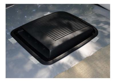
Before you start the next step, realize that the trim ring is 'sensitized' with the glue accelerant. Touching that surface with the tape means it will stay there. PERIOD! No, you CANNOT pull it off and reposition it. Touch it and it stays, like the guy in the commercial that glues his hard hat to the I-beam and then hangs from it. BE VERY CAREFUL in the next few steps!!!
