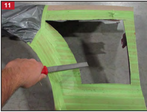
STEP 11: Use a metal file to remove any loose metal shavings or the lip that was created during cutting.
