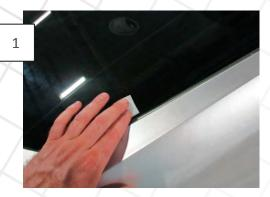
Using the supplied alcohol prep pads, wipe down the outer edge of the glass where the brackets will adhere. Once the alcohol has dried on the glass, repeat this process using the included 3M Adhesion Promoter.
