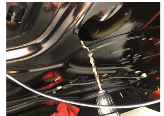
Step 8\\ Enlarge only the holes on of the structural skin. **Note: Drill slowly so that the drill bit does not make contact with the top of the hood. Drill a 17/32" hole so that the washer and phillips screw can pass through and sit flat on the underside of the hood skin.
