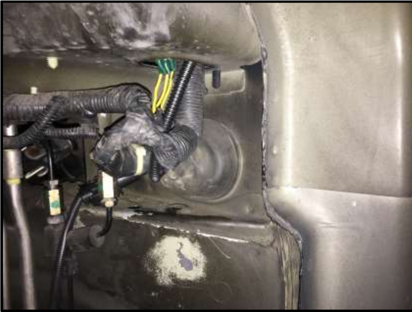
Figure J – Cable Routing through Engine Firewall and Up Into Engine Compartment
