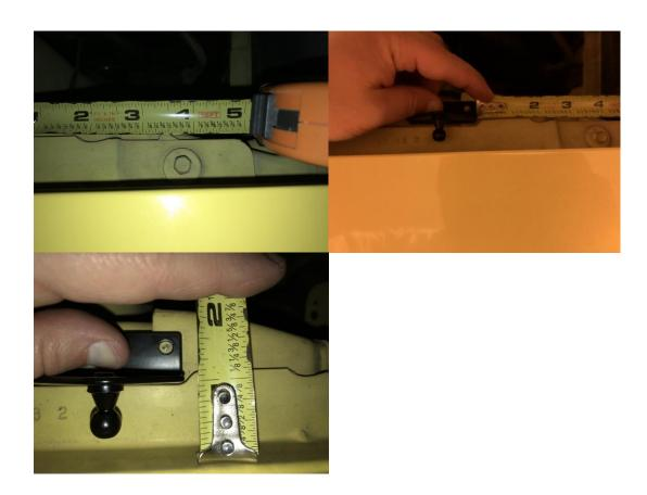
13. With the bracket in place, mark the first hole. Center punch the permanent marker to keep the drill bit from wandering like before. Drill the hole straight down using the 5/32" drill bit.
