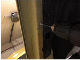
6. Test fit the bracket and one of the 4 shorter rivets (the two longer rivets are used for the center holes), if the rivet doesn't fit in just right you may ream out the hole slightly with the 3/16" bit.
