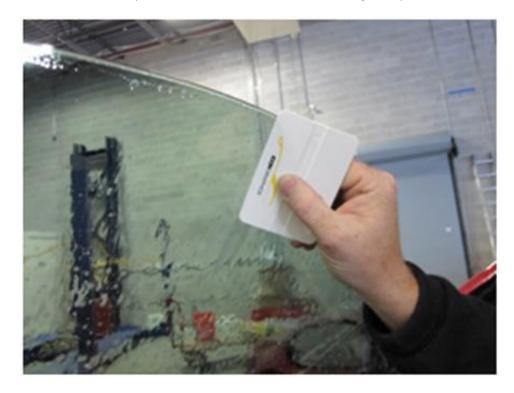
5. Using one of the supplied stuffer tools (whichever one fits your application the best), carefully tuck the tint into the rubber window trim as shown.
