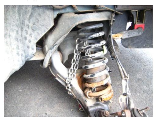
24. Transfer the old spring isolators, or use new ones if bought, to the new spring, and place the spring in the control arm. There will be two holes at the bottom pocket of the control arm, the pigtail needs to be in the middle of these two holes. So that it is covering one but not the other.
