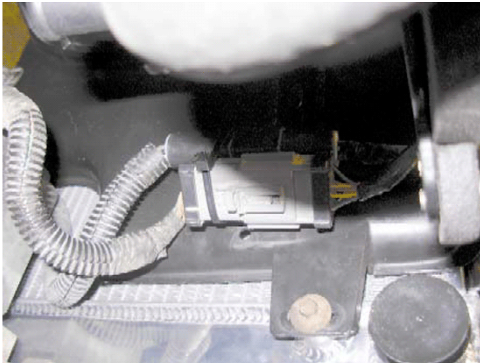
ABS connectors attached to fan shroud (looking down from above).
